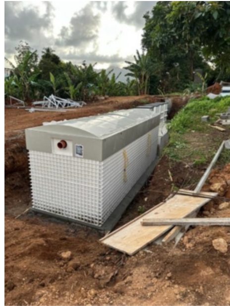
Aeration Tank installed on concrete pad
