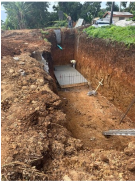
Concrete pad laid by NAWASA contractors for supporting the septic tanks which were imported from Edinburgh, Scotland .
