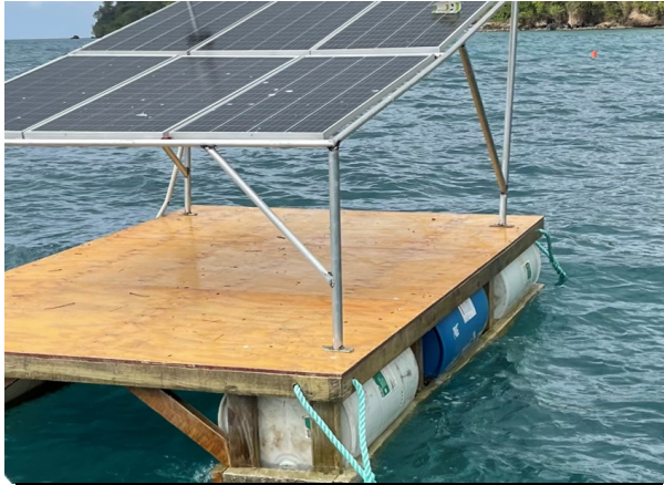
Figure 13: Coral Reef Restoration Programme Biorock technology component - floating solar panels, powering the Biorock coral reef structures
