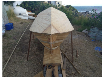
Figure 21: The bulbous bow under construction in Petite Martinique, Grenada
