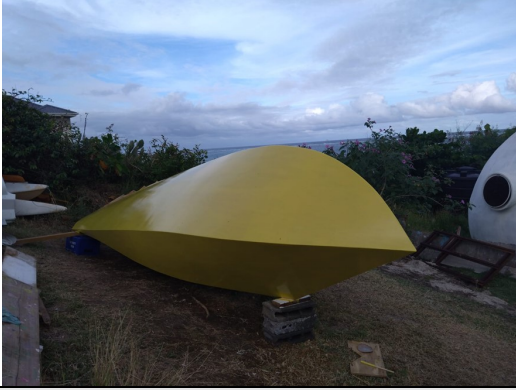
Figure 22: The bulbous bow under construction in Petite Martinique, Grenada
