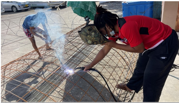
Figure 14: Coral Reef Restoration Programme Biorock technology component - community members welding structural components for the coral nursery
